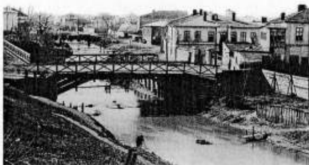
adu Vodă Bridge Photographer: Franz Duschek
